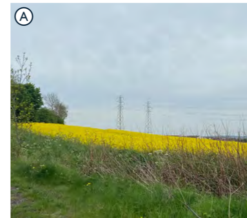
There are pylons and power lines running through the north of the site.
