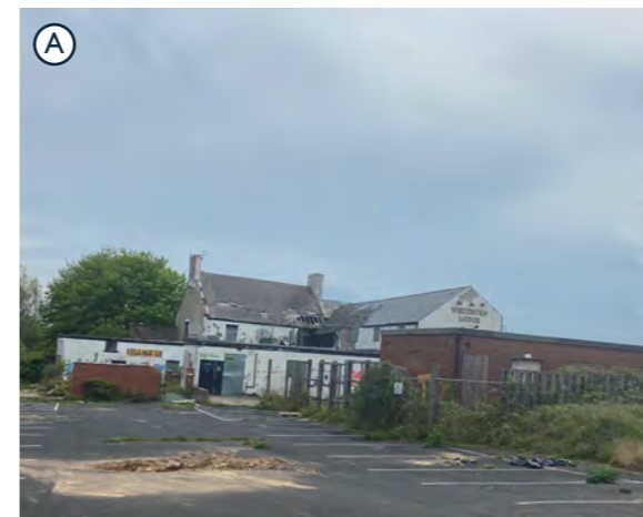
There are existing buildings on the site which will need to be demolished.
