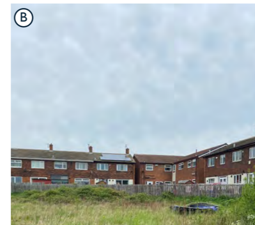
Existing houses back onto the site, and the area has been used as a fly-tipping location.
