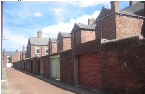
Original walls and openings remain largely unaltered.
