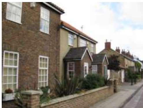
Nos. 40-42a Front Street succeed in echoing the modesty of the adjacent vernacular.
