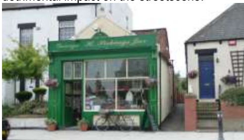
The village butcher's shop is one of the earliest buildings in this part of the street. It has changed little over the last 150 years and makes a significant contribution to the local scene.
