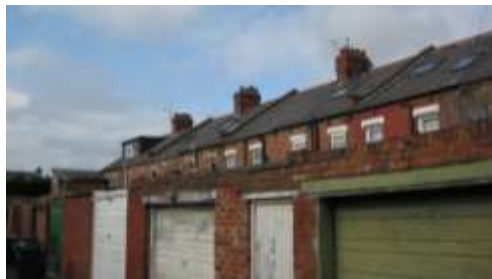
Small incremental changes, such as the introduction of dormers to otherwise intact roofscapes, can dilute the special qualities of a Conservation Area.
