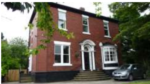
Shadwell Towers appears on the Local List. Placing it under an Article 4 Direction would give added protection from loss of features such as the original sash windows at ground floor level.
