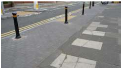
The large variety of unfamiliar materials fragments the streetscape. A plethora of bollards only adds to the overall street clutter.
