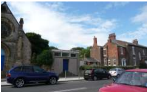
The design of this infill building has had a detrimental impact on the streetscene.
