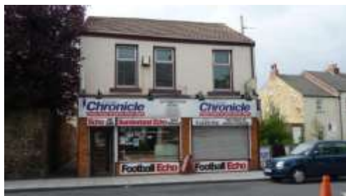
Unsympathetic alterations to this property include a modern shopfront with intrusive signage.
