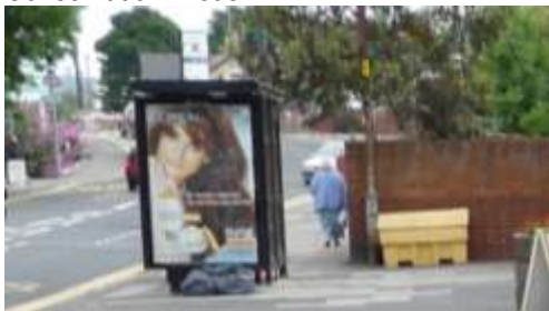
This bus shelter outside Station Terrace incorporates obtrusive advertisements.
