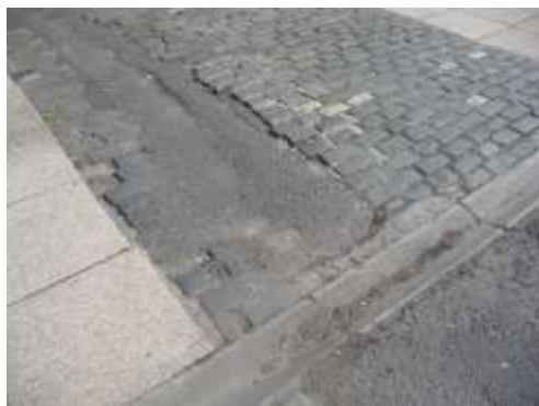
Several site accesses along Front Street have natural stone setts. Utility companies should be required to repair such surfaces on a like for like basis.
