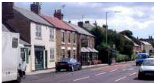
Character Area 1 represents Front Street, which forms the historic core of East Boldon.
