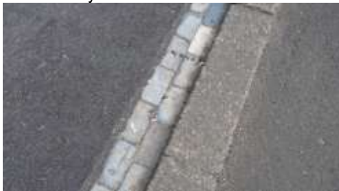
These traditional Scoria blocks along Station Road should be retained.
