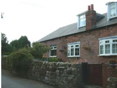
Sample of Quay Corner Avenue housing
