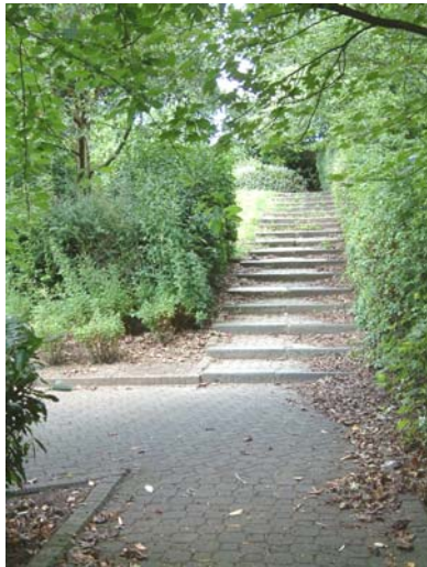
Path and stair detail within Drewett's Park
