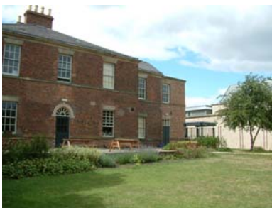
Jarrow Hall, east elevation and garden
