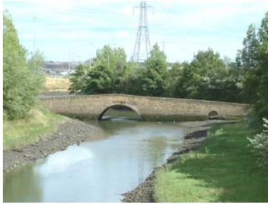
Jarrow Bridge, view looking east
