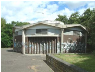
Don Valley Sewage Pumping Station
