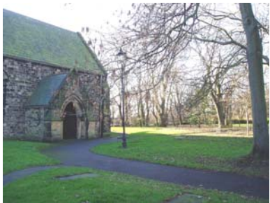
St. Paul's Church, north side and churchyard
