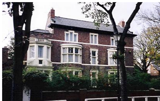
The Chase, no.19 (listed Grade II and covered by an Article 4 Direction, see 14.3) has been substantially altered over many years
