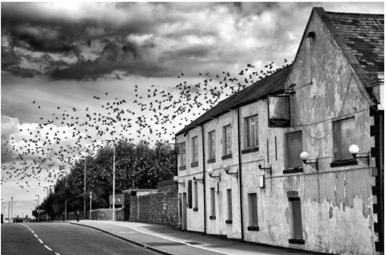
Figure 26 Whitburn Lodge. Photograph by John Short
