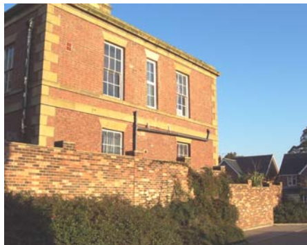
Alansway Gardens has significantly impacted on Westoe Villas
