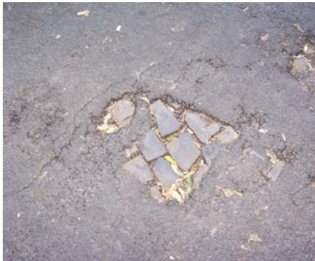
Original setts remain beneath later road surfaces
