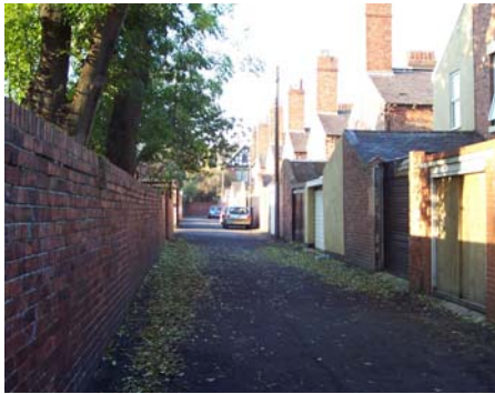
The rear of Village Terrace has retained its original built form nature
