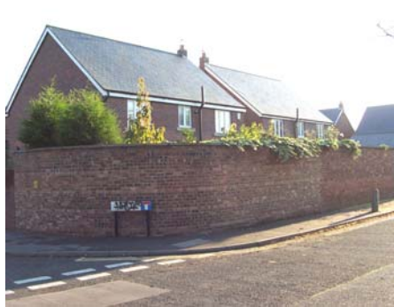
Alansway Gardens is an insular development and turns its back on Wood Terrace
