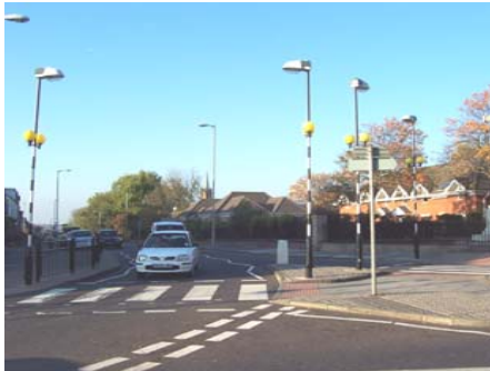
Road markings and signage can dominate the urban landscape
