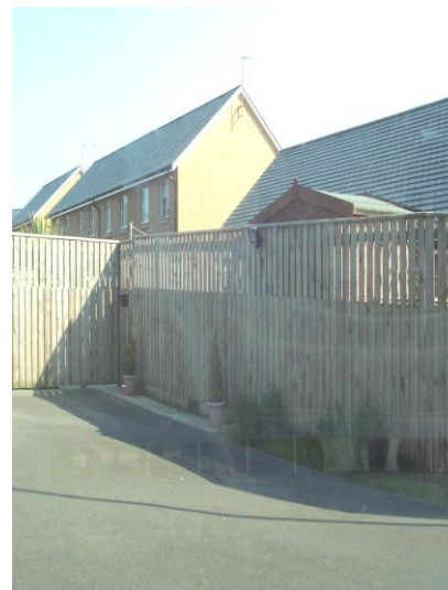
Cleadon Park – rear fencing
