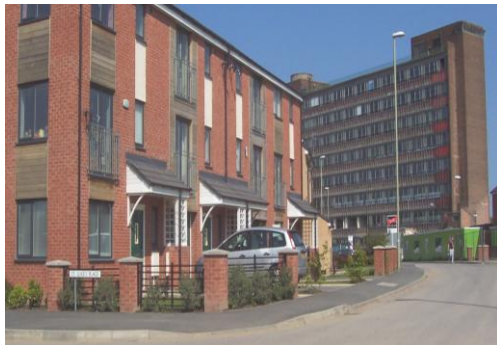
Boundary Treatments at Riverside Park, Hebburn
