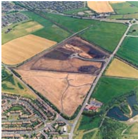
Monkton Cokeworks Reclamation, Hebburn Business park development site incorporating new community woodland and a network of strategic and local recreational routes
