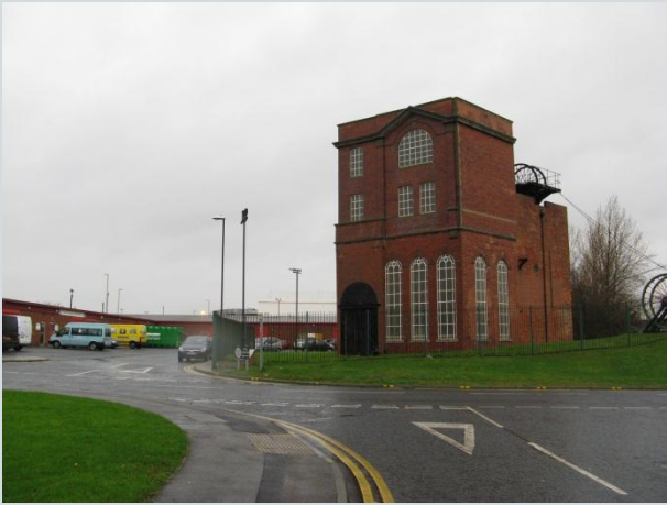
Preserved building of St Hilda's Colliery
