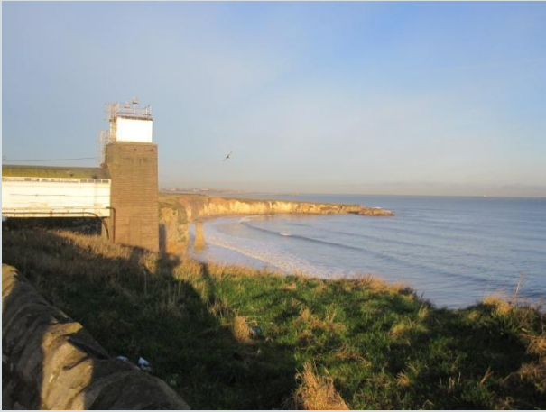
Lift shaft at Marsden Grotto
