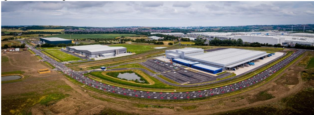
Figure 1 New Buildings and Access Road at IAMP ONE
