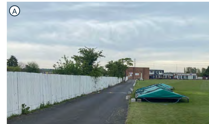
Boundary to the neighbouring sports facility.
