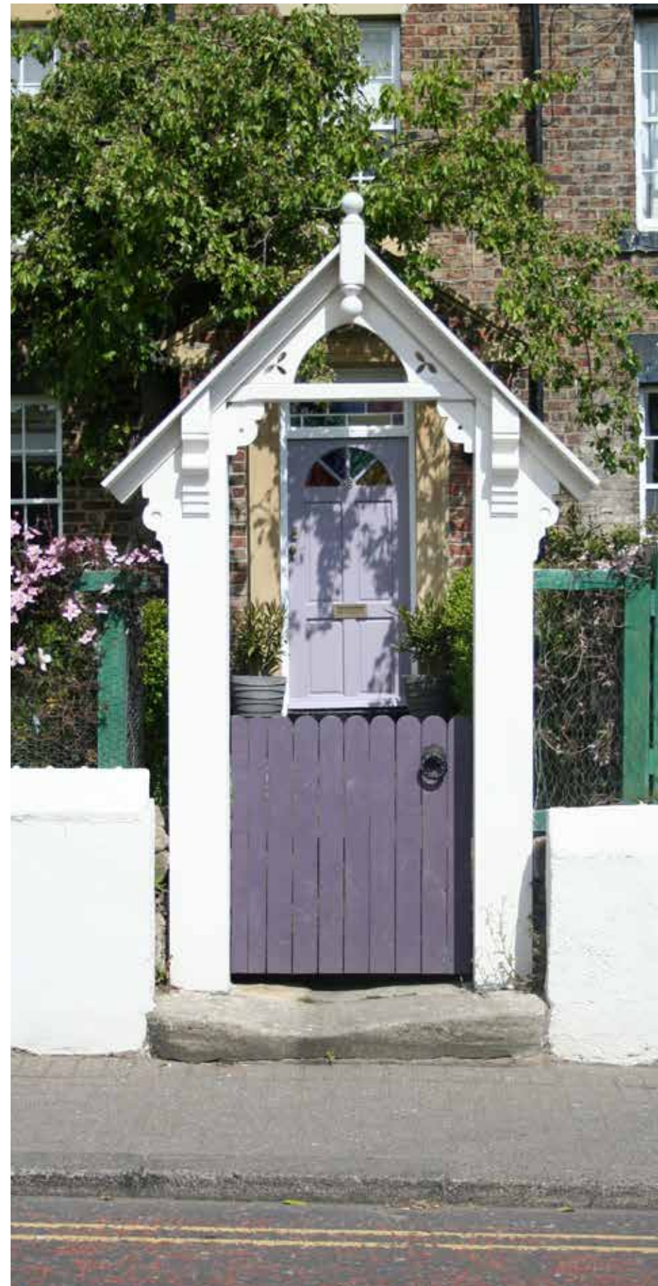
The entrance to Nos.33 and 35 (Pear Tree Cottage), North Guards
