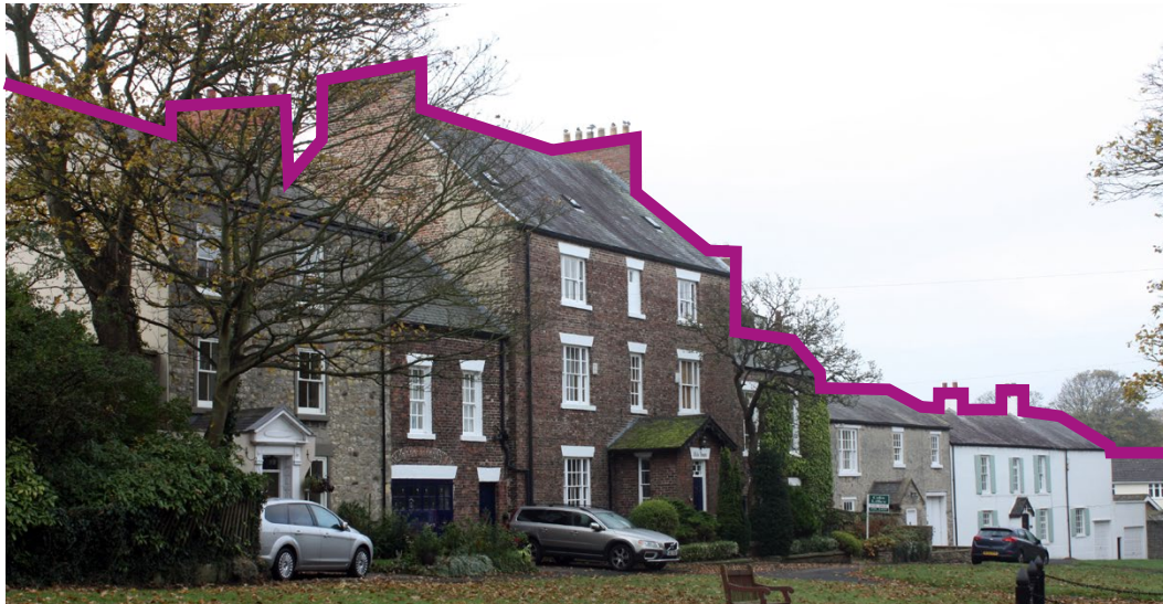
Figure 17: Local example showing rooflines with variety
