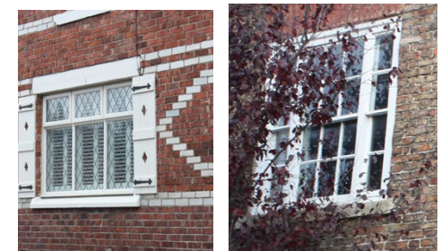
Figure 39: Casement window details
