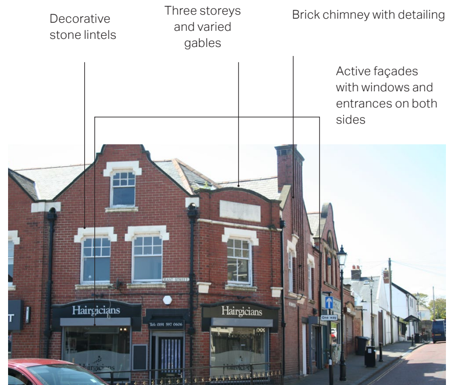
Figure 20: Local example showing a traditional treatment of a corner building
