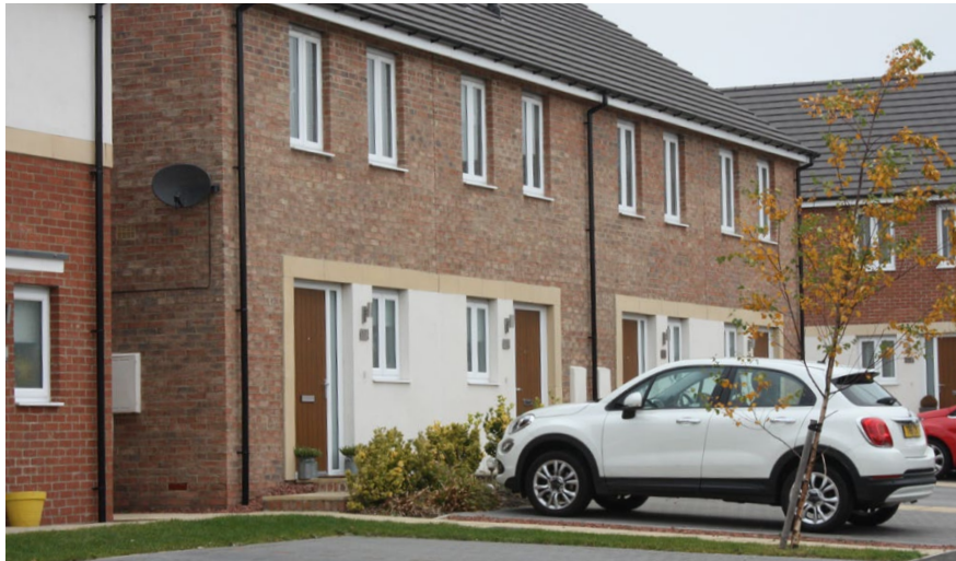
Figure 21: Local example of car park arrangement, treatment and detail
