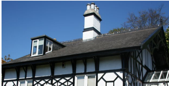
Figure 33: Varied Dormer windows
