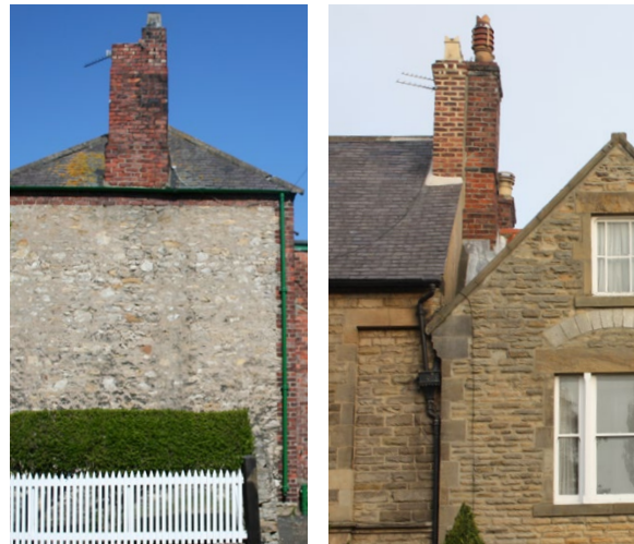
Figure 35: Brick chimney on hipped and gable roofs
