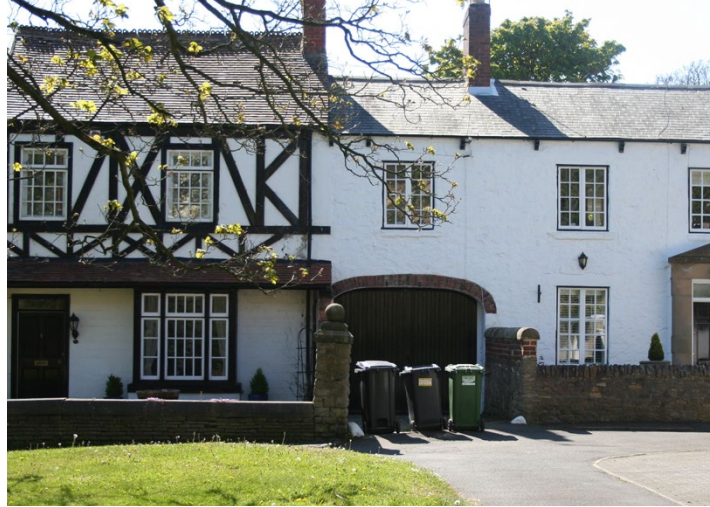
Figure 28: Typical architectural building with white painted stone, timber frame, and high quality details on rooflines, gutters and boundaries
