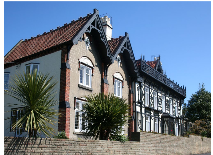
Figure 25: Deep eaves and carved bargeboards on Whitburn House and Lodge
