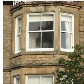
Figure 40: Typical bay windows
