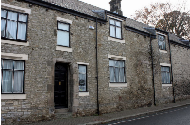
Figure 27: Local example of traditional architecture with buff stone work, stone lintels, and casement windows.
