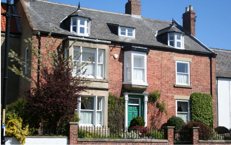
Figure 26: Brick facade and traditional windows with stone lintels, with decorative entrance and boundaries using brick and ironwork details
