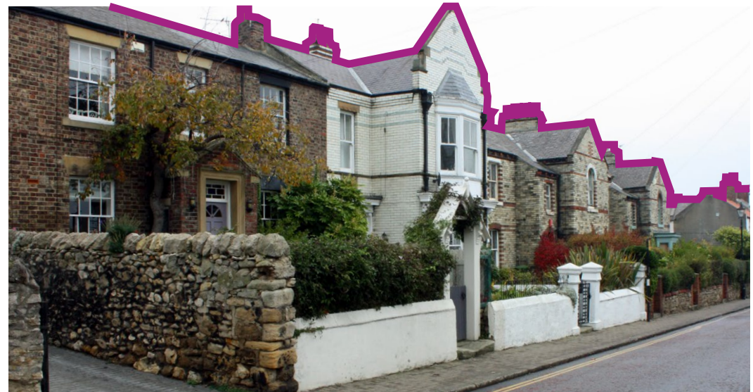
Figure 18: Residential roofline with variety and interesting change in topography
