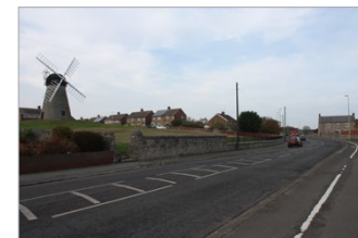
Mill Lane, looking north
