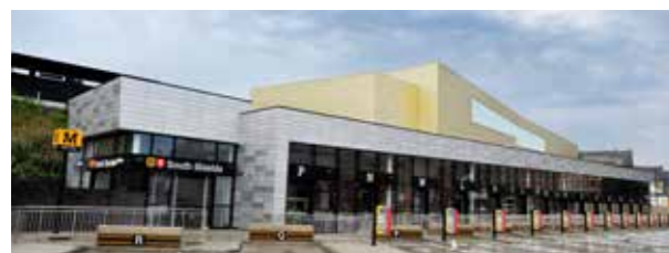
£21m South Shields Transport Interchange
