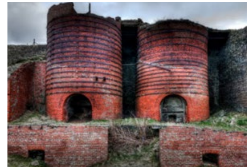
Historic Lime Kilns at Marsden
